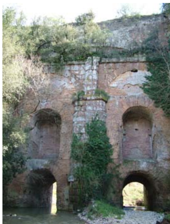
Figure 2 : The Aqua Marcia Lupo Bridge
