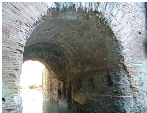
Figure 3 : The Lupo Bridge: horizontal layers, arches and intrados vault.
