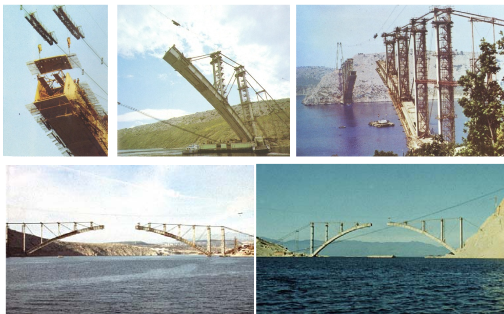
Figure 20: Photos of arch construction
